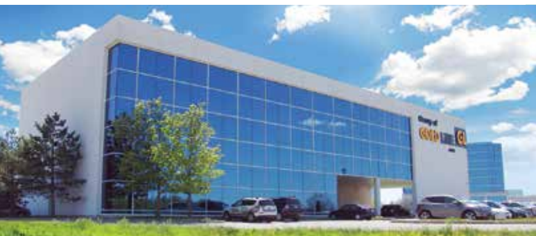
Gold Line's state-of-the-art Markham Data Centre is housed within the company's Canadian headquarters.
