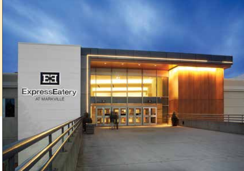
EXP has provided engineering solutions for Markville Mall's expansion, redevelopment and renovations for almost 20 years.
